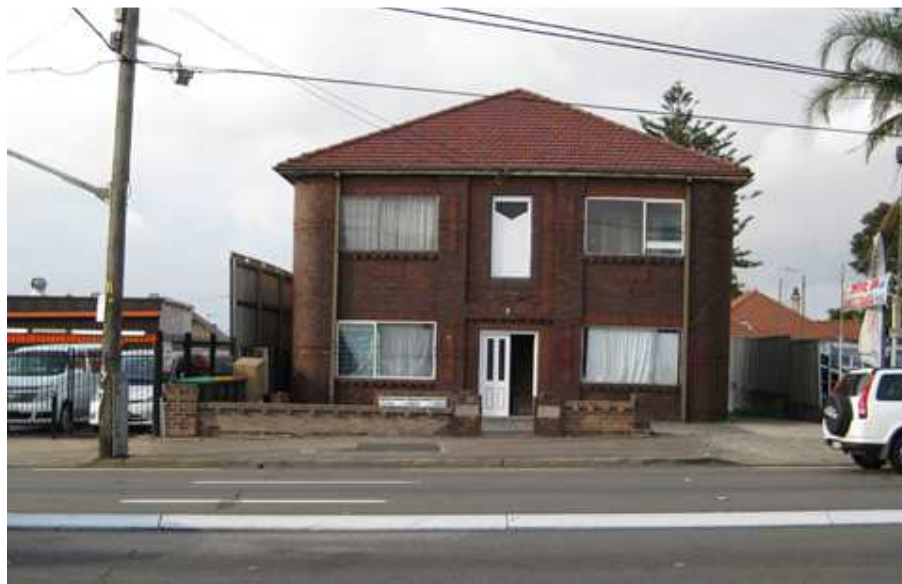
Figure 2 – Derelict property 69 Parramatta Rd.
