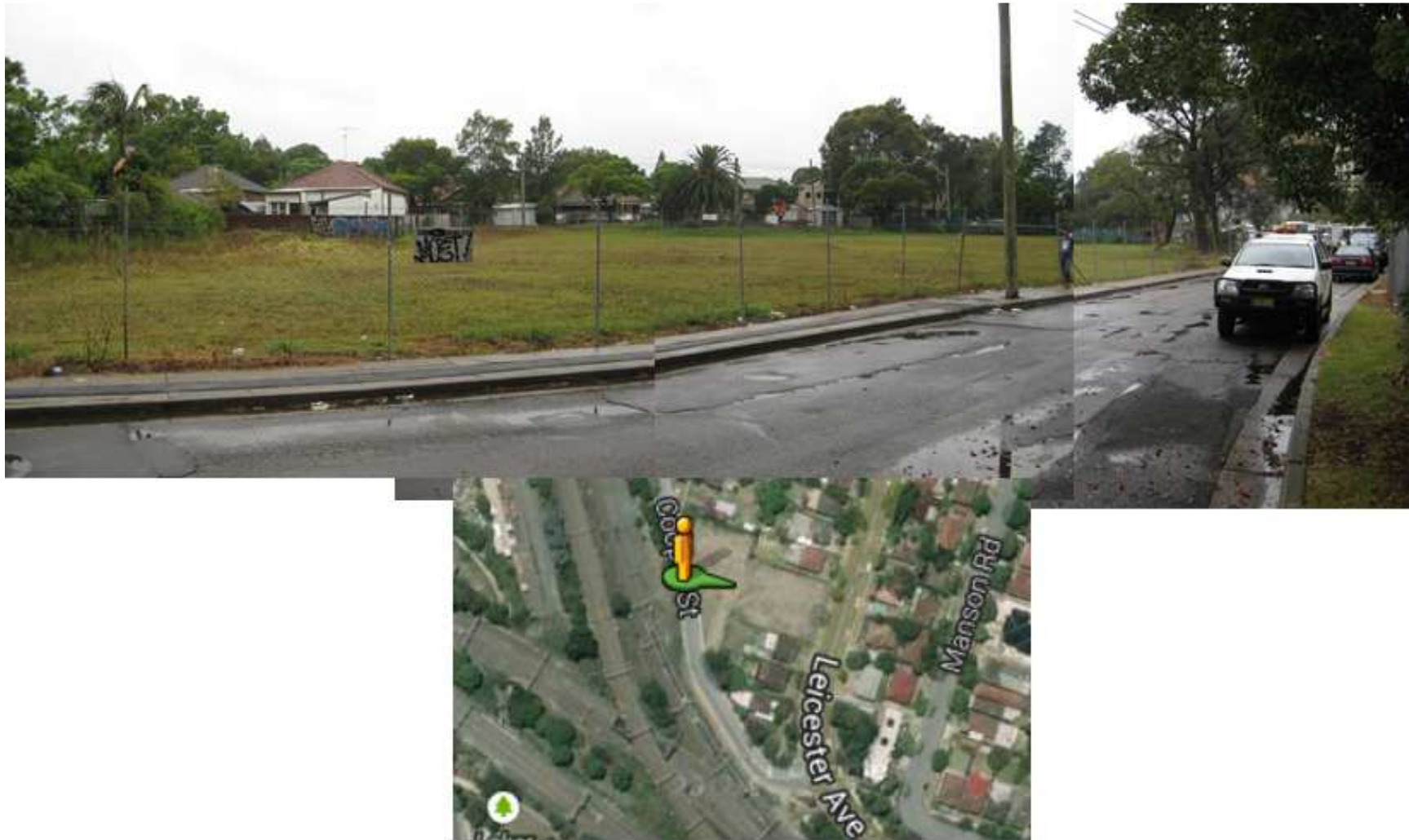
Figure 8 – View of ‘Strathfield Triangle’ development area taken from Cooper St looking toward Leicester Ave.
